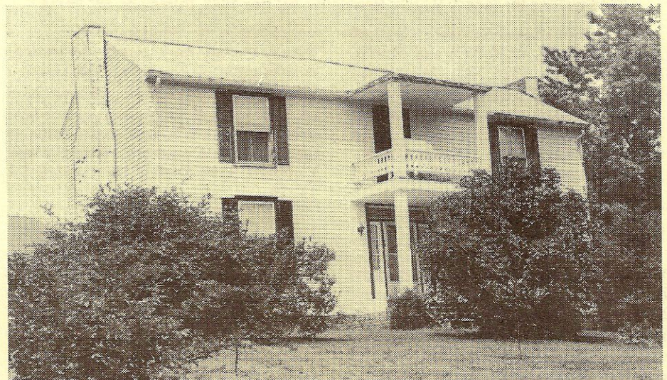
Stabilization work will begin soon on the museum house in preparation for restoration, which will be done in several phases. When completed, the museum will be an important step in preserving Yancey's history and culture.
